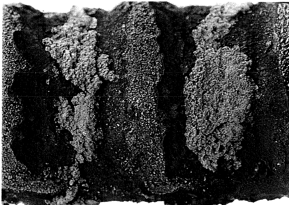
Photo 5.14. Close-up picture of a corroded surface showing various types of corrosion products.
