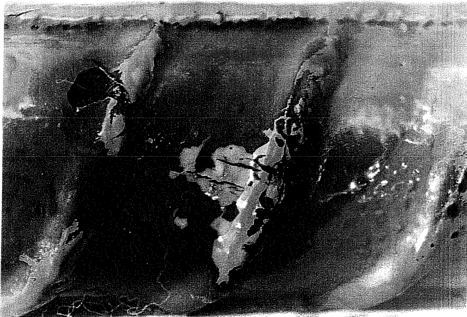
Photo 5.43. Close-up picture showing cracks formed on a patched ECR specimen after immersion in 3.5% NaCl solution for 200 days.
